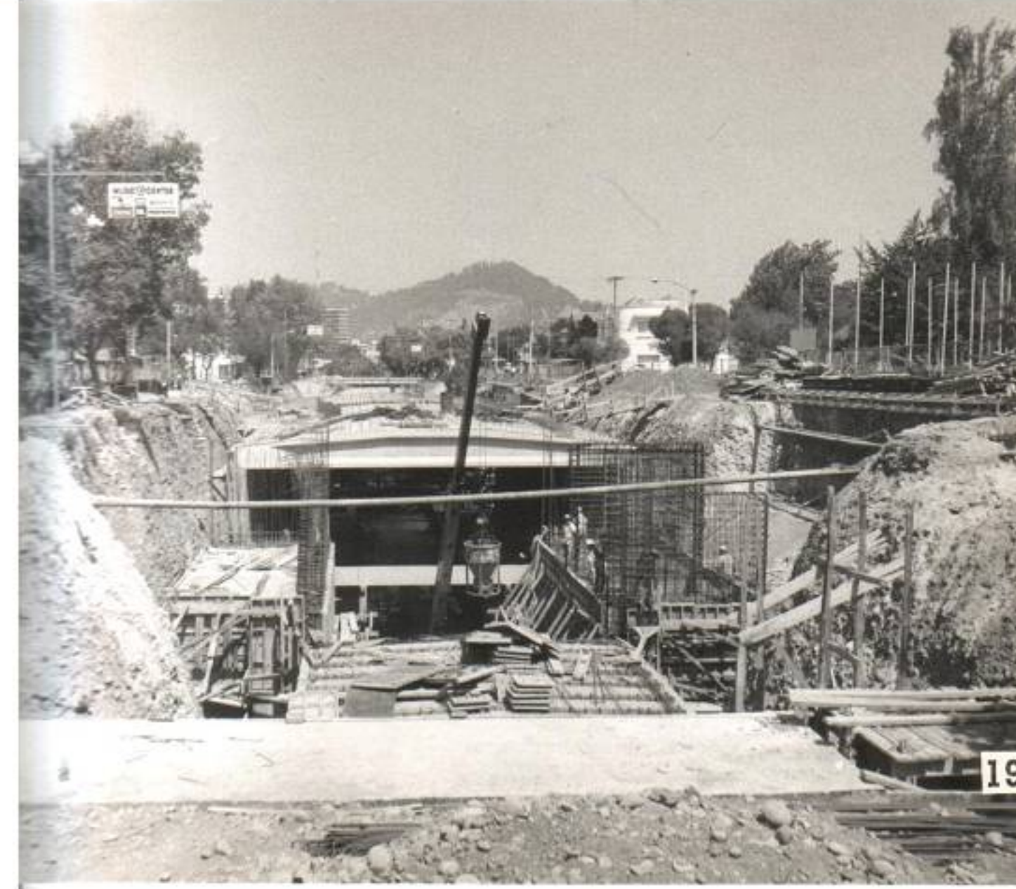
Line 1 - Station El Golf
