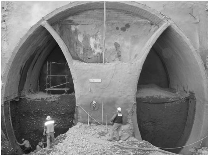
Figure 4. Double side wall drift station excavation.
