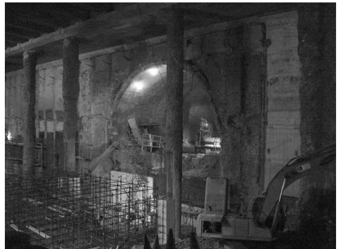
Figure 7. Quinta Normal Station excavation.
