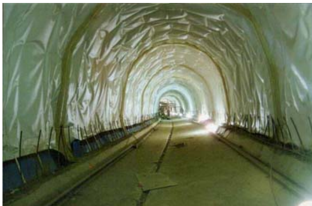
Figure 28a: Membrane waterproofing used on Section F6b WMATA - Washington, DC 1995
