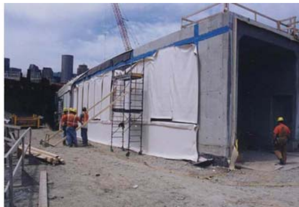
Figure 28a: Membrane waterproofing used on Section F6b WMATA - Washington, DC 1995
