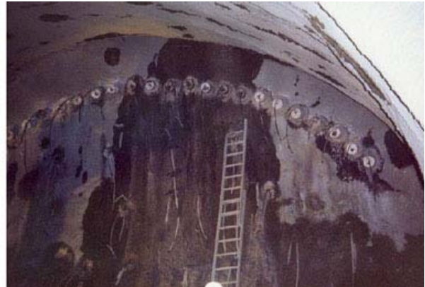
Figure 10b: Grouted pipe spiling installation at tunnel face Monastiraki Station - Athens, Greece 1995
