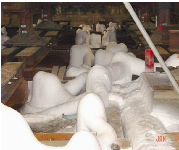
Figure 19a: Freeze pipes in basement of Russia Wharf Building above tunnel MBTA – Boston, MA 2002 Figure 19b: Tunneling around an obstruction and timber piles in frozen ground MBTA - Boston, MA 2002
