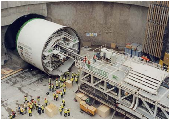
Figure 1a: TBM launch at Dublin Port Tunnel - Dublin, Ireland 2002
