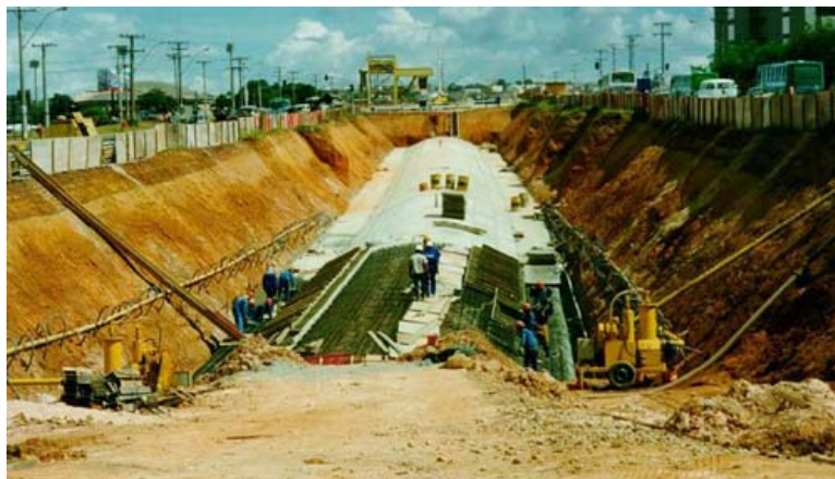
Figure 23: DFM installation at Taquatinga Metro Tunnel - Brasília, Brazil 1995
