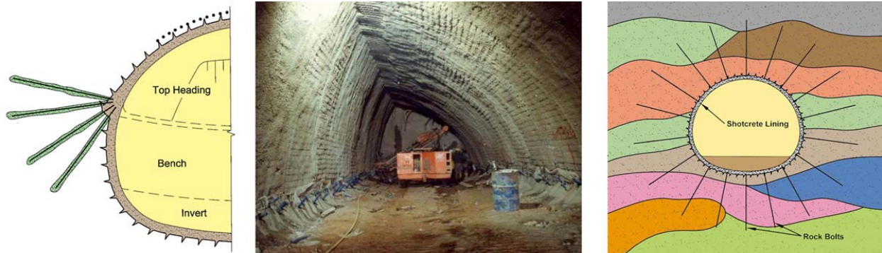
Figure 17a: Grouted spiles at sidewall footings.
