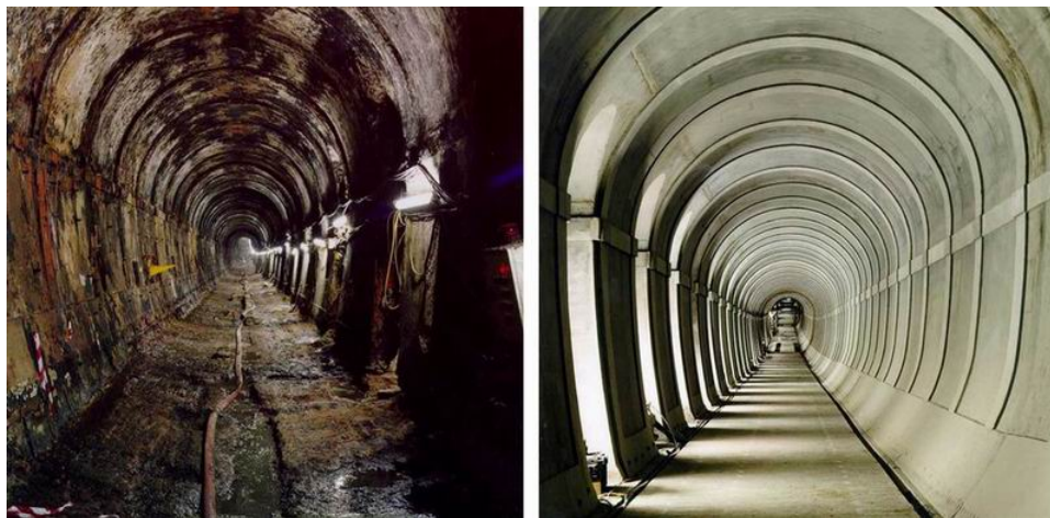
Figure 30a: Brunel Tunnel constructed beneath the Thames River in 1830's LUL - London, UK 1995
