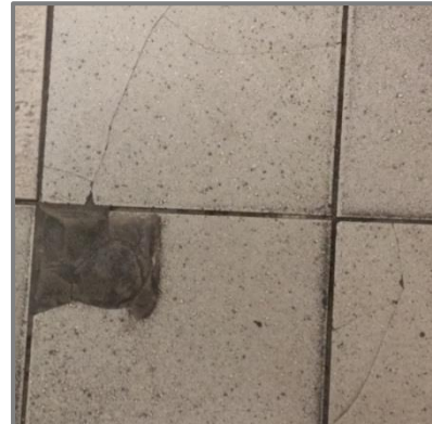
Tiles cracked/broken at the floor
