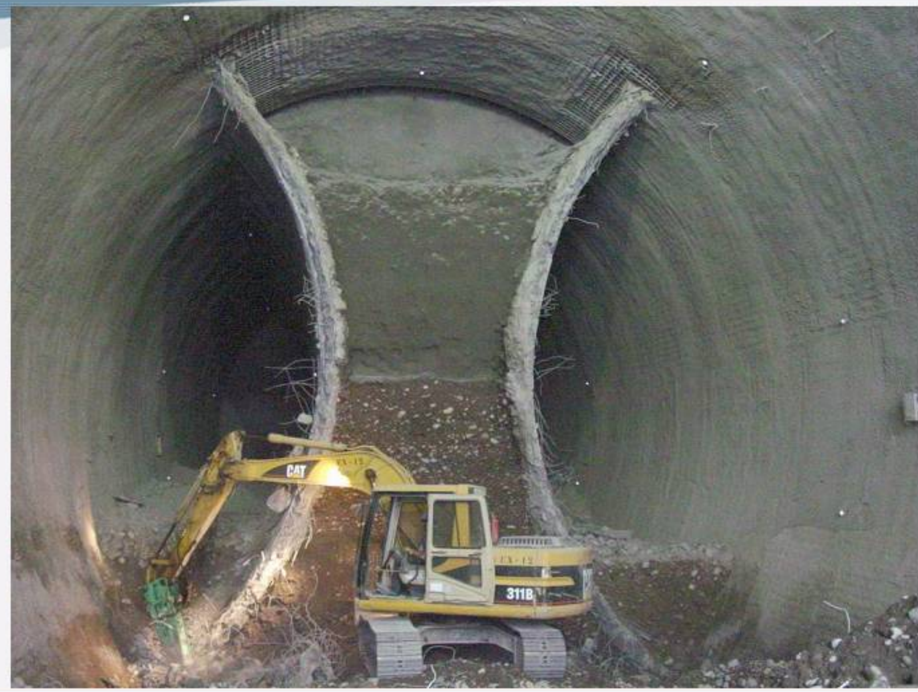
NAT 2004 - Atlanta, GA Beacon Hill Station, Seattle, WA
