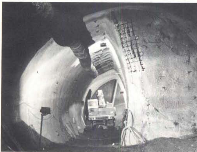
Excavation of the first sidewall drift of the Type 2 sequence.
