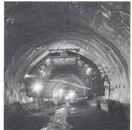
The form for the purpose of installing the membrane.
