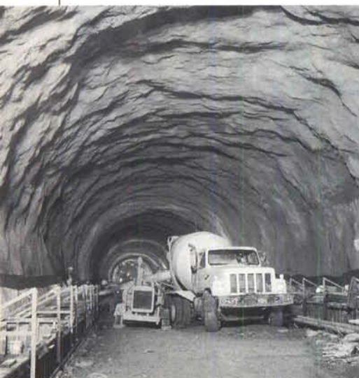
Tunnel with shotcrete.
