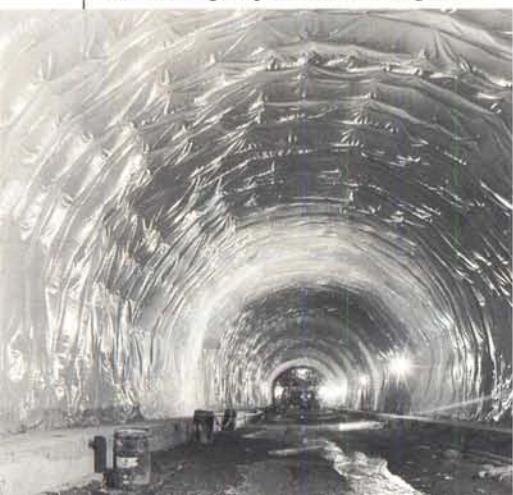
PVC waterproof membrane in place.
