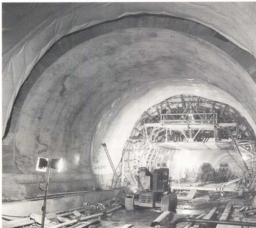
Final lining and the slip form.
