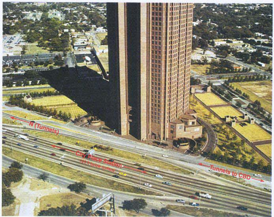
Cityplace location and North Central Expressway. Cityplace Station will be located 120ft beneath the North Central Expressway with connecting passages to the highrise buildings above.
