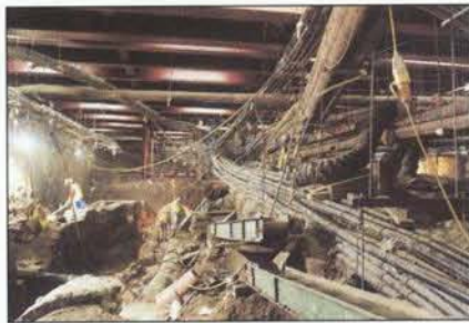
Covered excavation of the ticket hall beneath Borough High Street.
