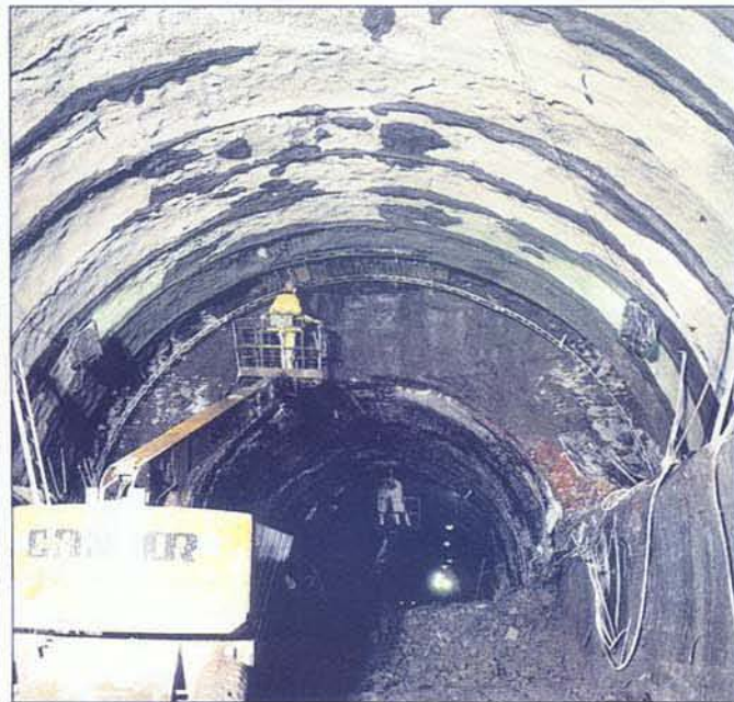
Erecting Pantex lattice girders as the existing tunnel section is enlarged.
