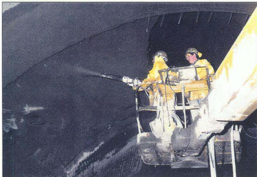
Shotcreting for support.
