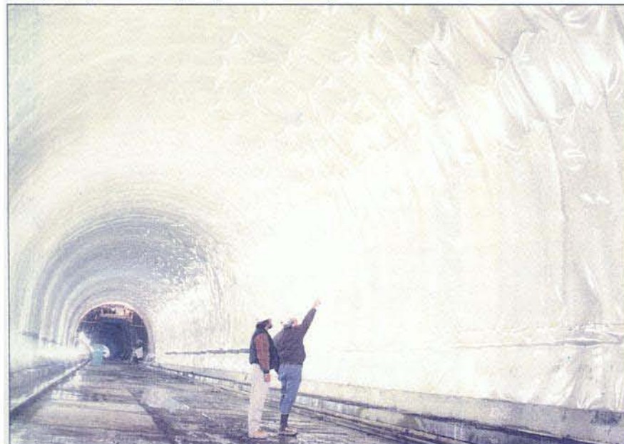
Waterproofing membrane in place prior to final lining.
