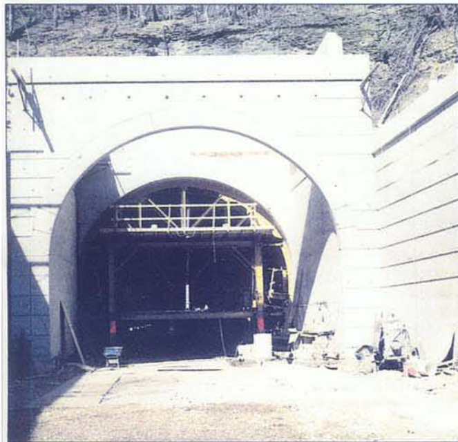
Berry Street portal with concrete formwork in position.
