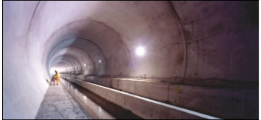
North Downs tunnel, recently completed and ready for track laying.
