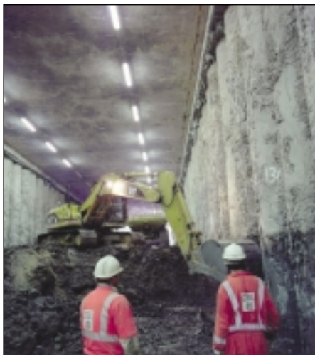
Left: Boxley tunnel showing bored piles.
