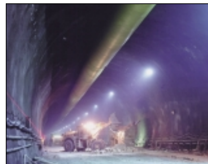
Construction in the North Downs tunnel.
