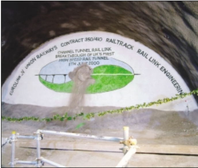
North Downs tunnel – initial roadheader breakthrough in June 2000.
