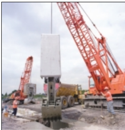
Digging the diaphragm well for the Stratford Box.
