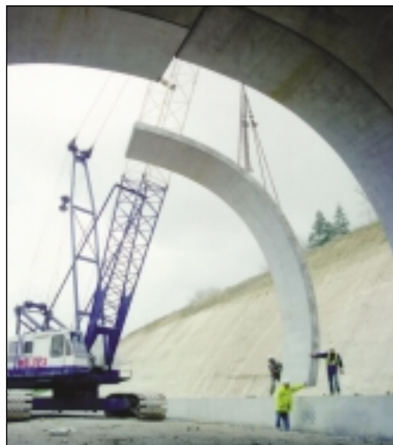
Right: Cladding placement at Eyhorne tunnel.
