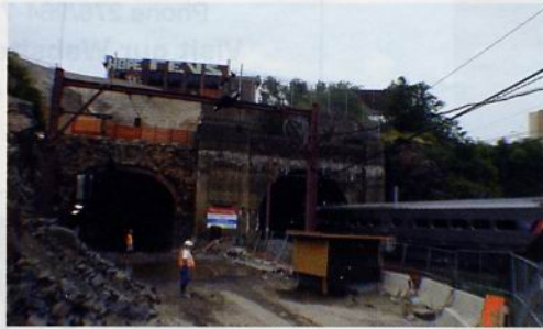
Rehabilitation of the oldest of two Bergen Tunnel tubes.
