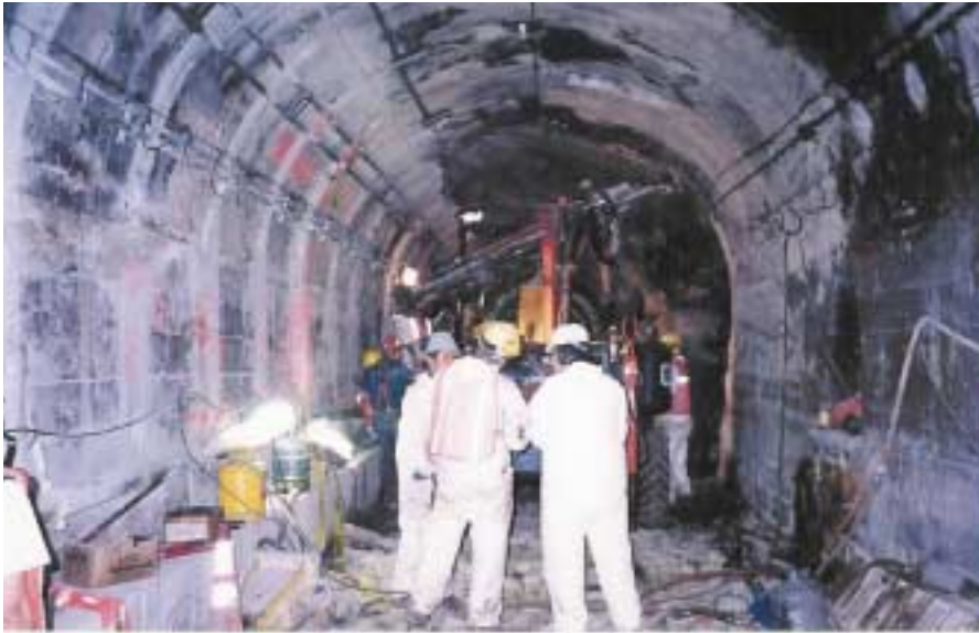
Beginning of tunnel excavation
