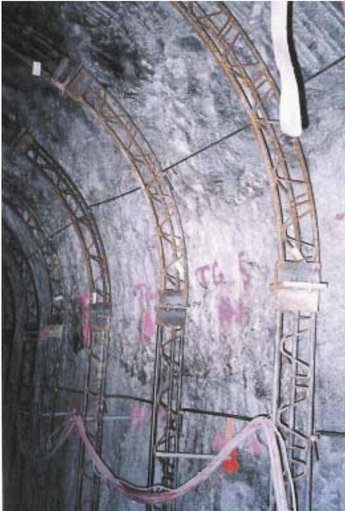
Some of the lattice girders specially designed for the project
