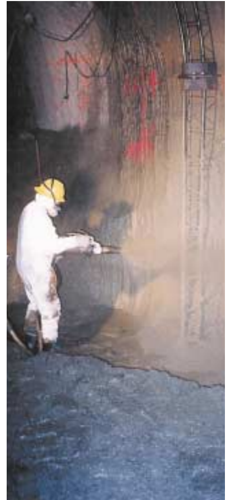
Shotcrete application over lattice girders
