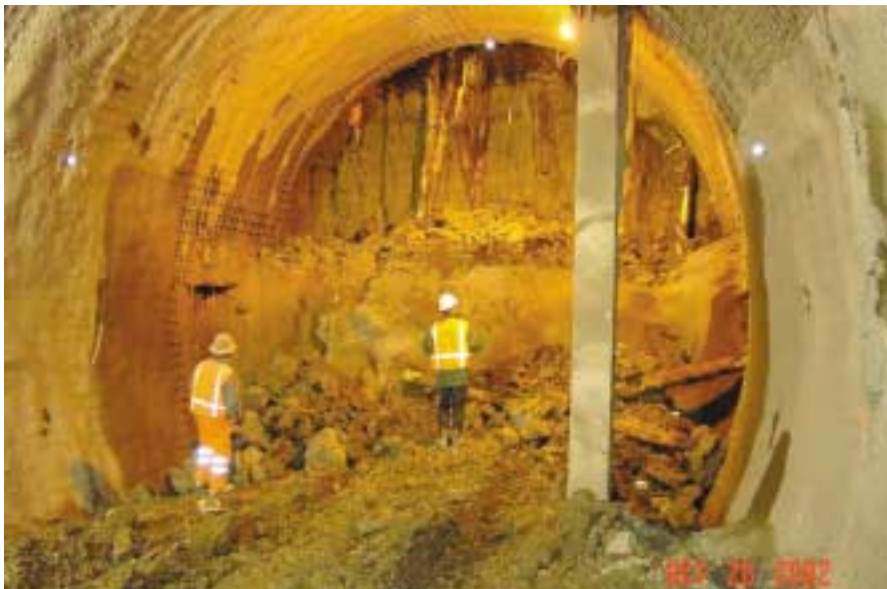
Tunnel excavation showing wooden piles in the working face
