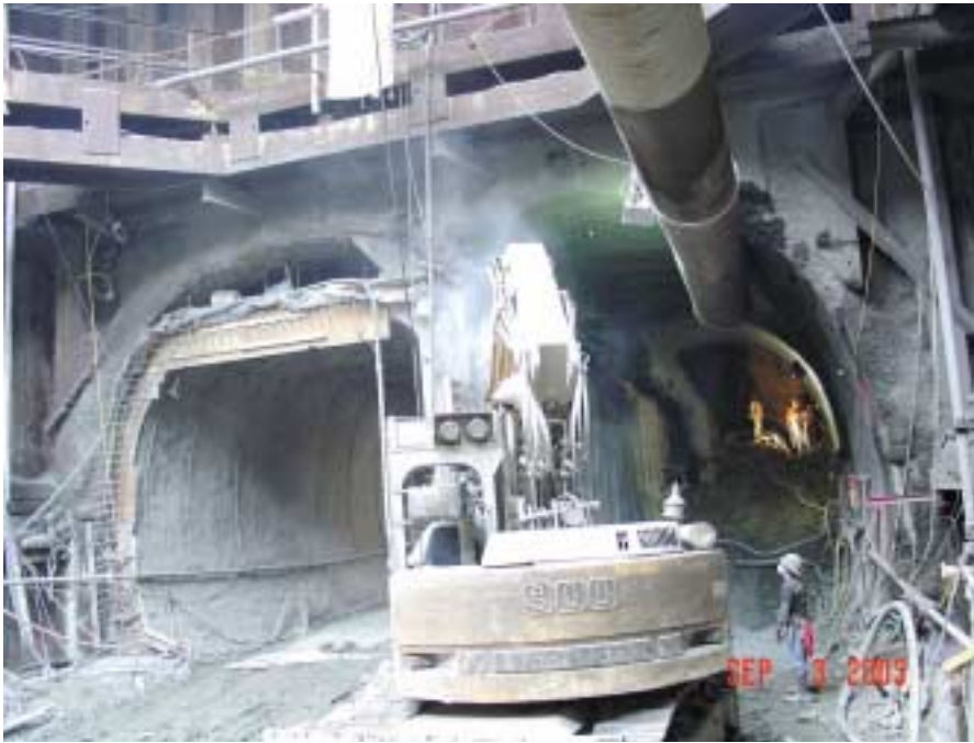
Tunnel portal view with Liebherr 900 excavator in foreground
