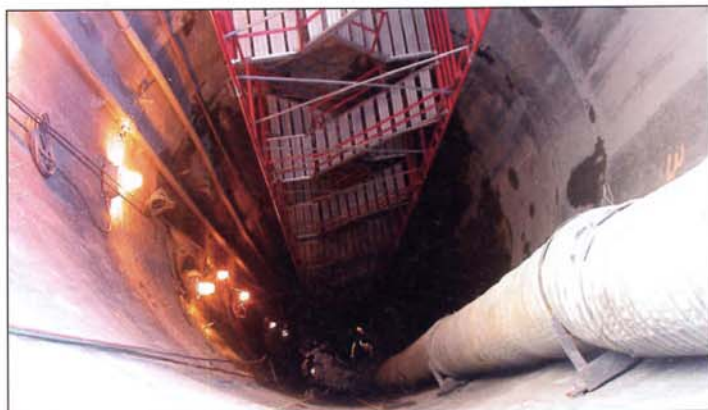
Interested parties were provided access to the test shaft construction
