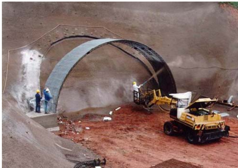
Figure 27: Shotcrete canopy portal structure at B27 Bypass Tunnel - Schürzeberg, Germany 1991
