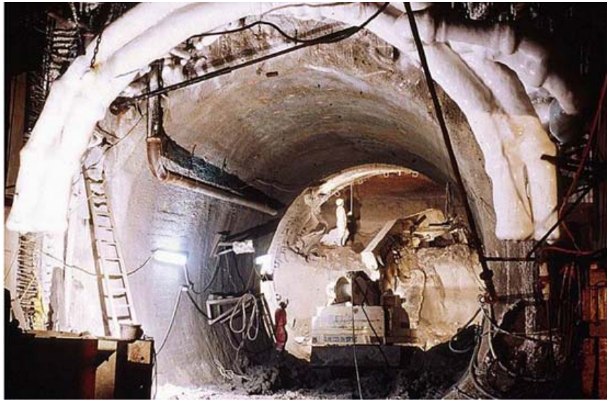
Figure 12a: Vertical freeze pipes above rail tunnel portal - Hannover, Germany 1985
