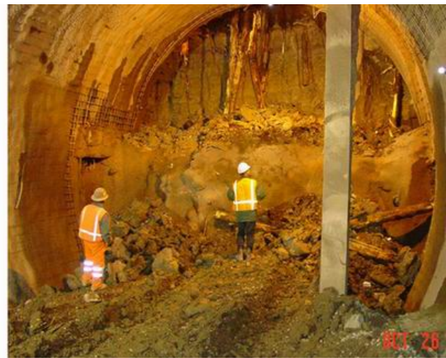
Figure 19a: Freeze pipes in basement of Russia Wharf Building above tunnel MBTA – Boston, MA 2002 Figure 19b: Tunneling around an obstruction and timber piles in frozen ground MBTA - Boston, MA 2002
