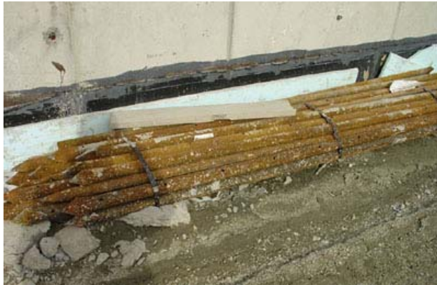
Figure 10a: Grouted pipe spiles MBTA – Boston, MA 2004
