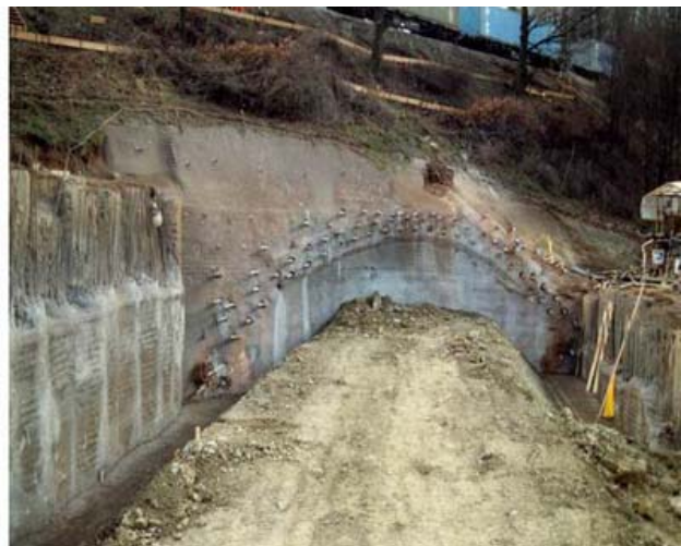
Figure 13b: Barrel Vault tubes installed beneath active rail line - Oberrieden, Germany 1990
