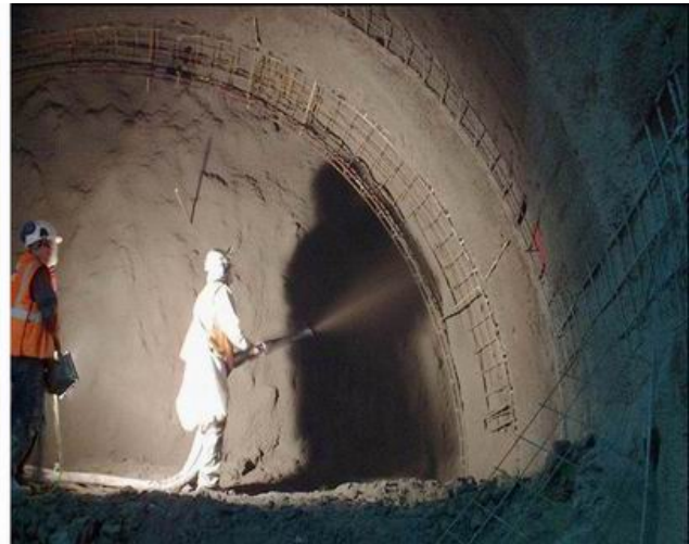
Figure 8b: Shotcrete application at top heading of Lehigh Tunnel #2 - Allentown, PA 1990
