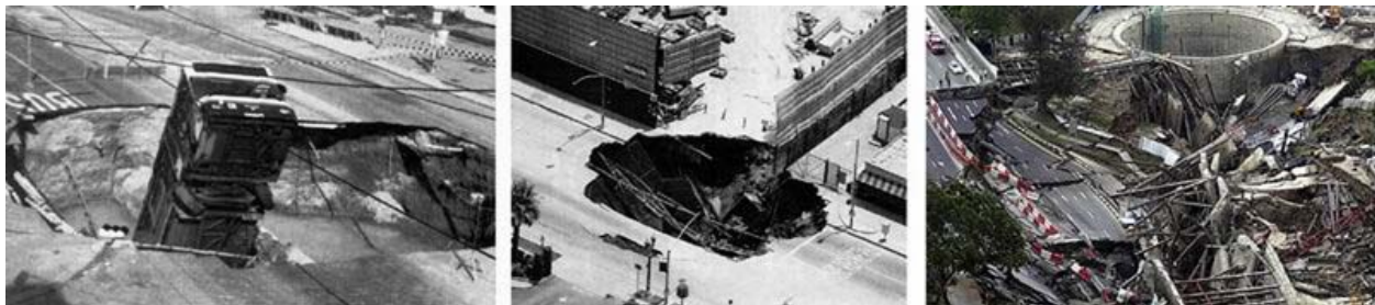
Figure 7a: NATM tunnel collapse on U-Bahn Subway - Munich, Germany 1994
