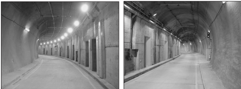
Figure 7. Finished inbound and outbound tunnels
