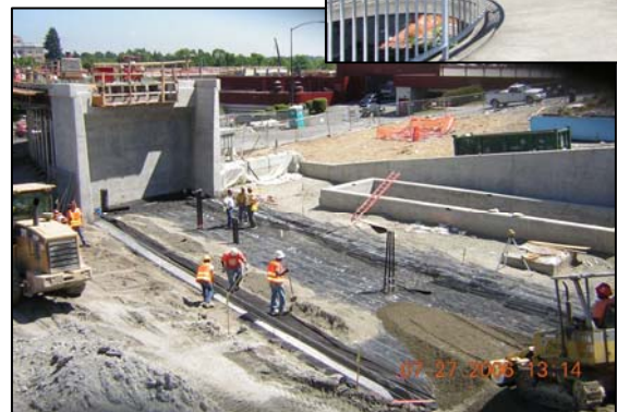
Starting to build the earth embankment at the east portal (below)
